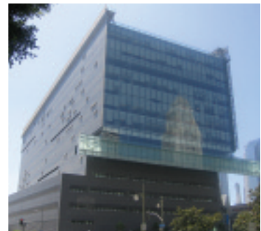
Caltrans District 7 Headquarters , Los Angeles, CA
